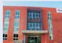
Peking, China ○ IGBT-Stack-Montage
